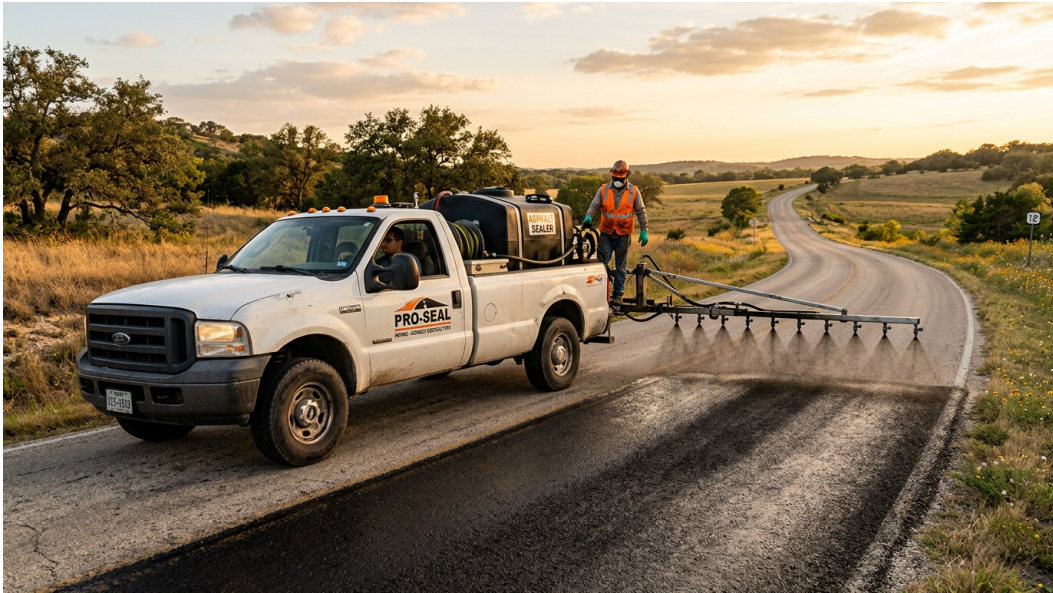
Boom sprayer applying HawkSeale solution to a road surface
