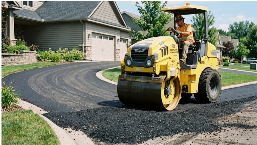
Ride-on roller compacting HawkSeale-treated millings
