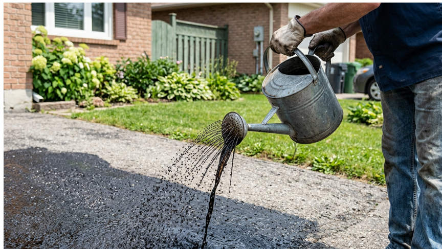
Sprinkle can with drilled holes for fan-like application
